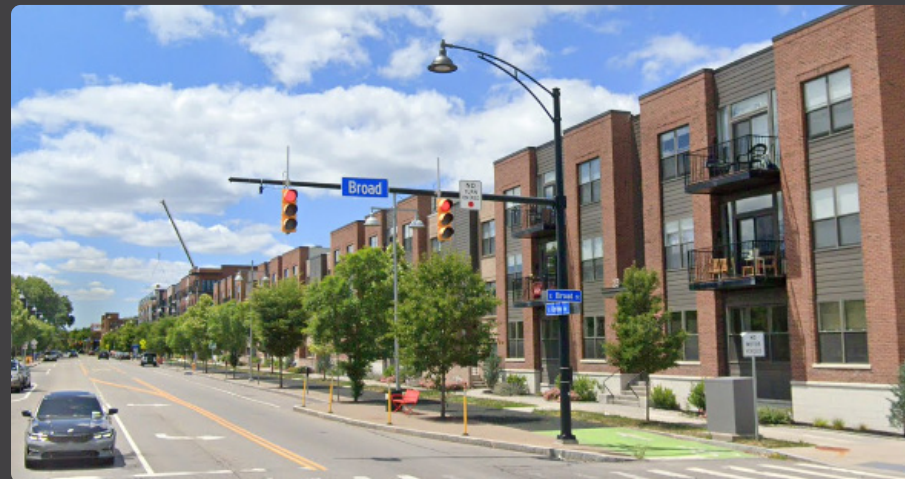
Union Street in Rochester, NY, former location of Inner Loop East Freeway. In the mid-2010’s, the City of Rochester and NYSDOT converted a sunken, obsolete freeway that divided the community into an at-grade complete street, promoting redevelopment and reconnecting neighborhoods with their downtown.
