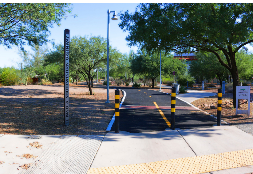
Off-street accessible trail with wayfinding signage, striping, lighting, and other amenities
