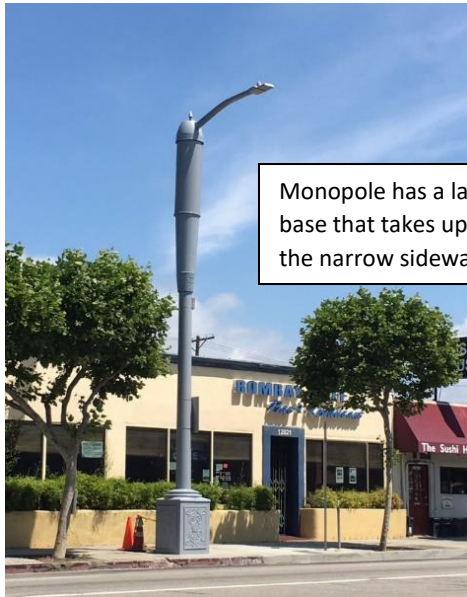
Figure 4-1: Unacceptable Monopole Installation
