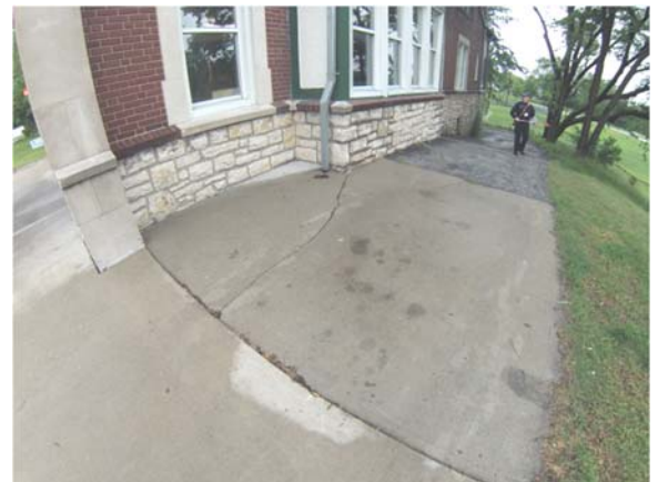
Damaged Concrete Driveway
