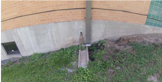
Downspout Erosion
