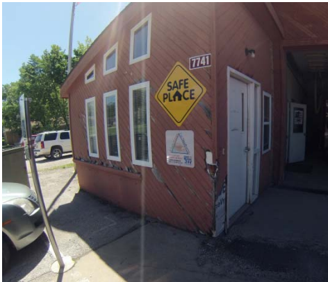
Front Entry Siding Damage
