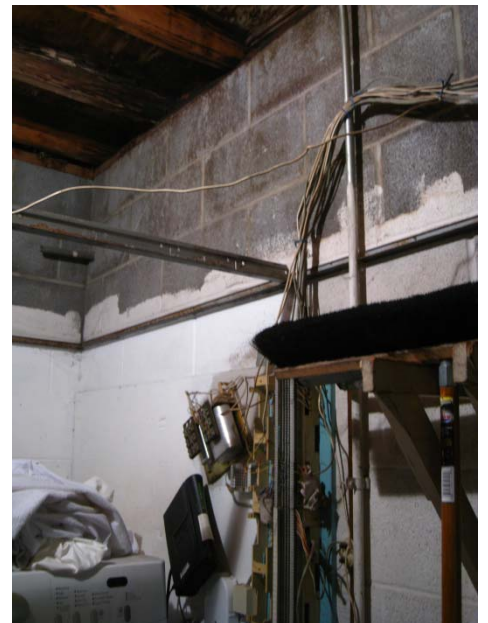
Roof Leak Over Phone Equipment
