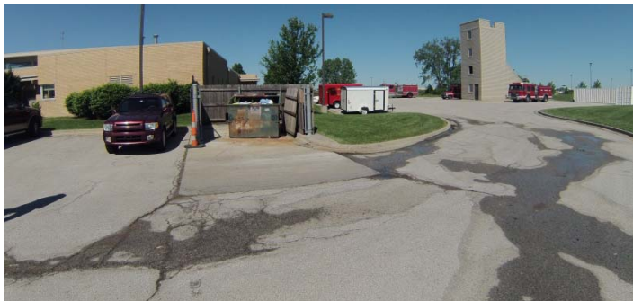
Parking and Drive Asphalt Deterioration
