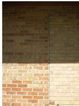
Cracks in Masonry
