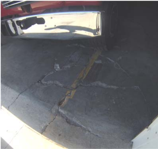
Significant Cracking in Bay Corner
