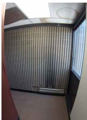
Scorched Wall at Radiant Heat
