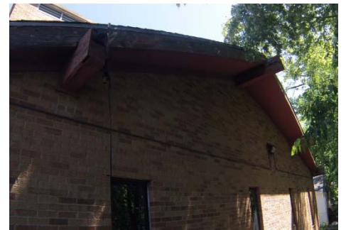
Rear of Station with Raw wood Beams and Fascia
