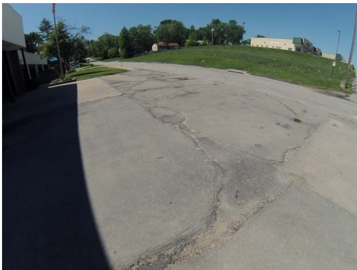
Front Apron Concrete Cracks
