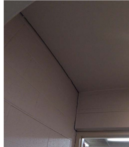
Large Crack in Hallway Masonry
