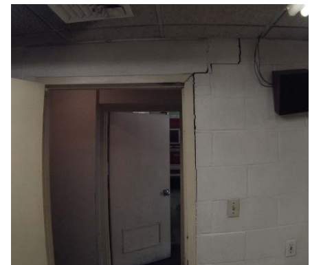
Crack from Bathroom Side of Hall
