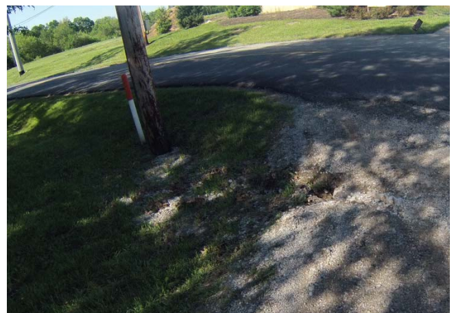
Crushed Culvert at Rear Drive
