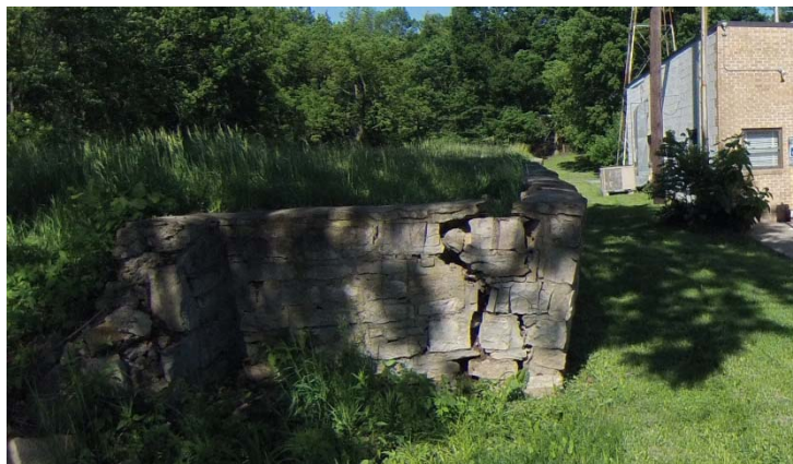
Structurally collapsing Retaining Wall
