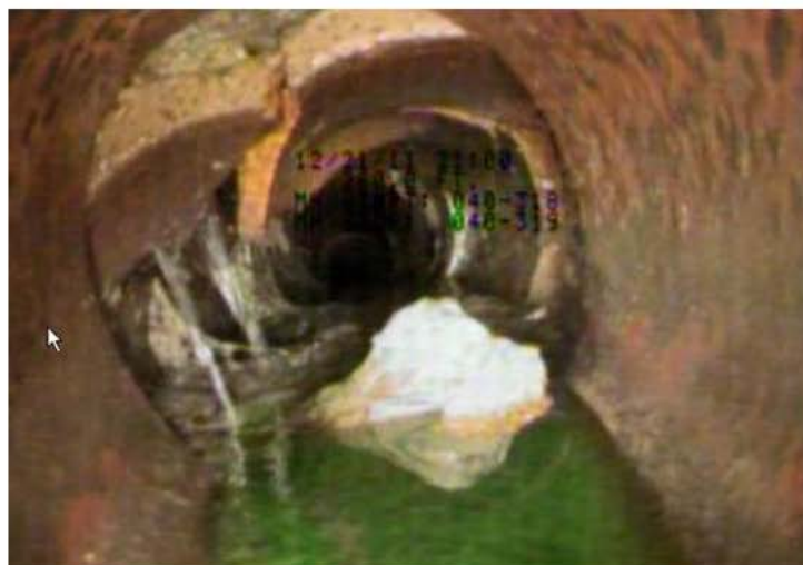
The UG experiences overflows due to various types of infrastructure failures, including collapsed pipe.
